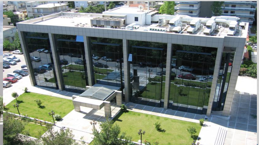
Office block in Halandri
