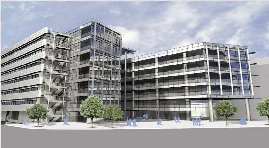
Building of office block in Kifissias Avenue (Athens)
