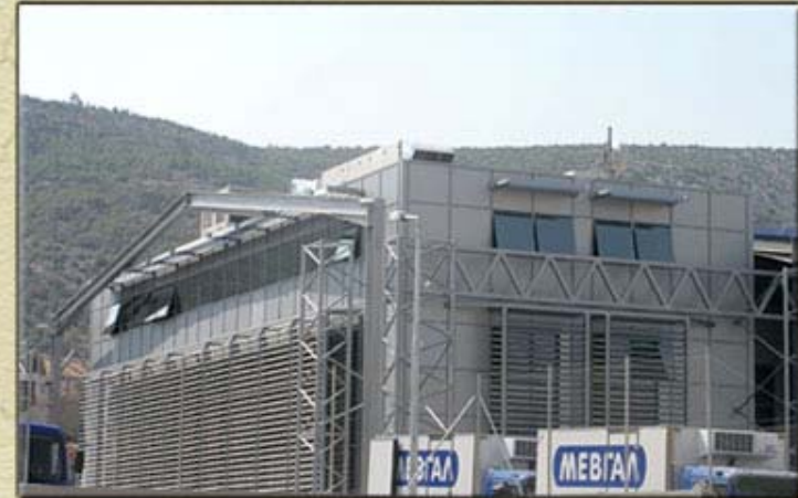
GREECE, PRODUCTION UNIT OF DAIRY PRODUCTS, M5600
