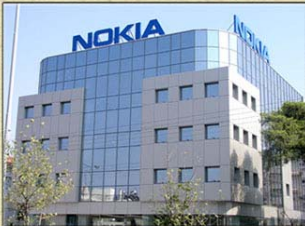
GREECE, NOKIA BUILDING, M4
