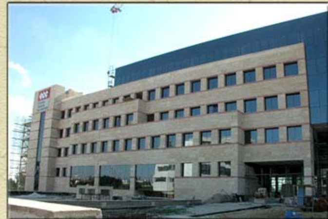
CYPRUS, ELECTRIC COMPANY BUILDING, M4, M9050
