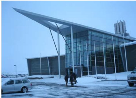
Geothermal power plant in Iceland
