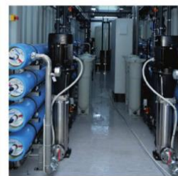
Figure 2: pressure exchangers reduce energy use in the RO booster pumps.
