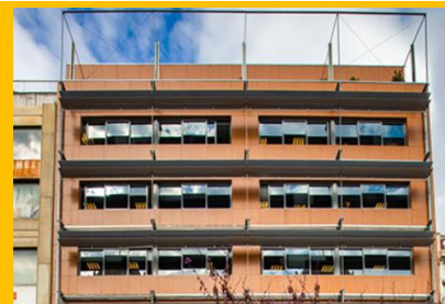
67, Aioulou Str, Athens Eight-storey building, 3.022 sqm
