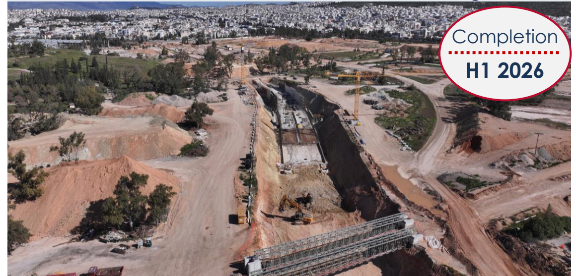
The Ellinikon Mall Underpass 47% of excavations and 10% of concreting
