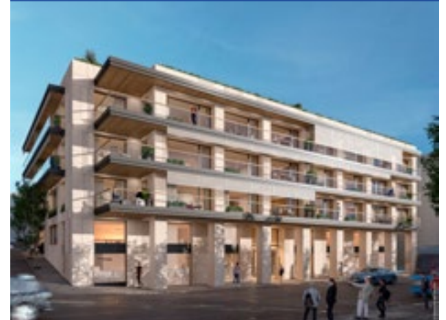
Mets Residential and Office Building
