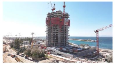
Concreting works: 17<sup>th</sup> level Core Structures & 14<sup>th</sup> level Slabs
