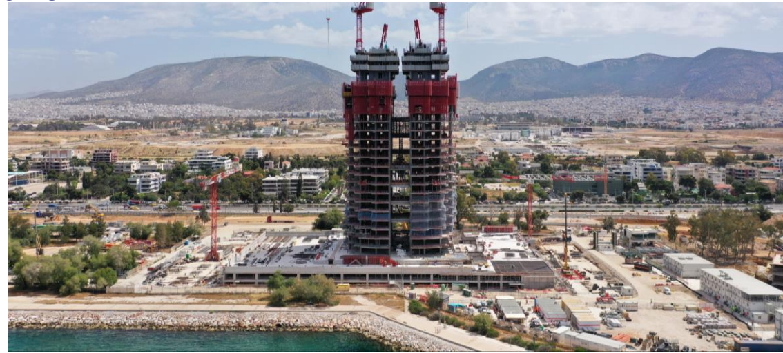
Concreting works: 21 st level Core Structures & 19 th level Slabs
