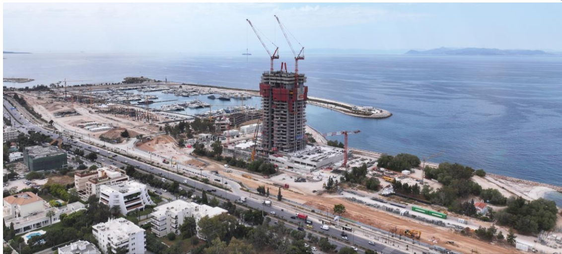
Concreting works: 21 st level Core Structures & 19 th level Slabs
