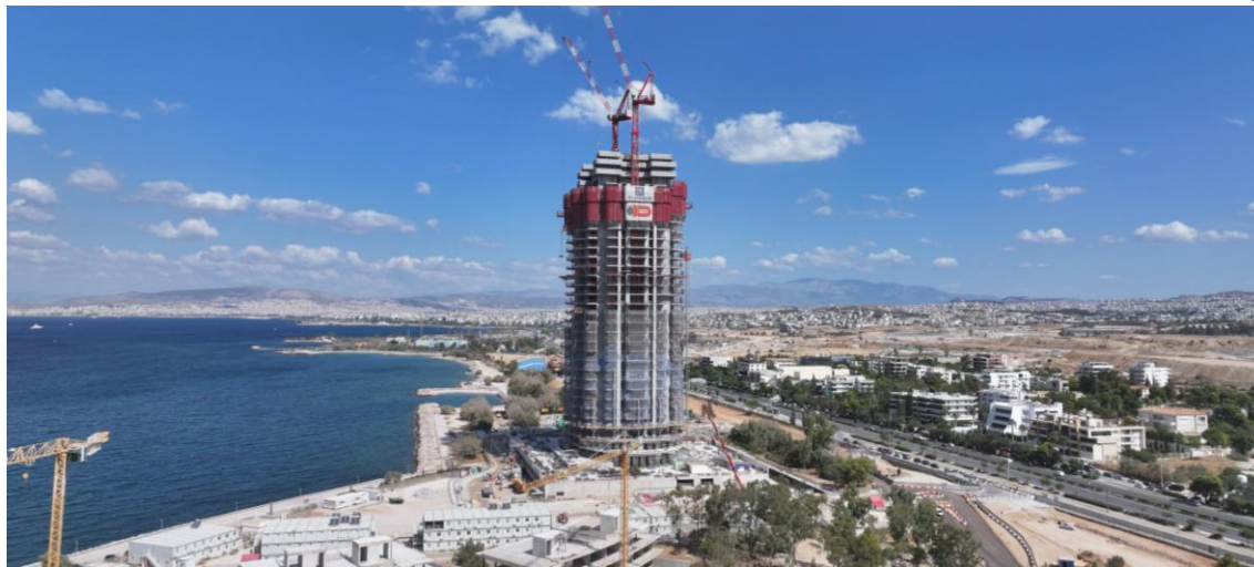
Concreting works: 31 st level Core Structures & 28 th level Slabs
