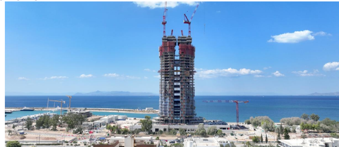
Concreting works: 31 st level Core Structures & 28 th level Slabs
