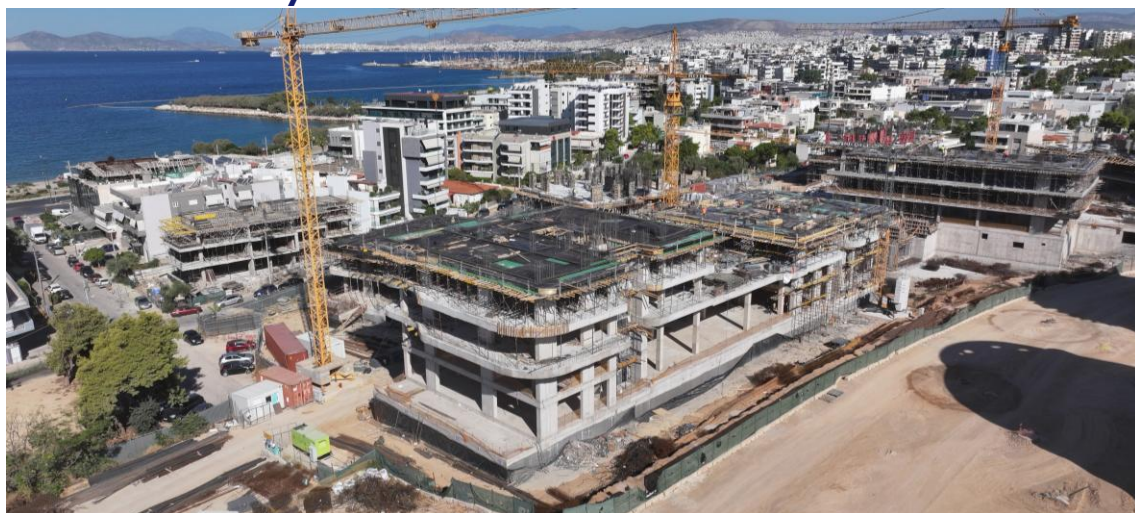
Superstructure concreting works in progress
