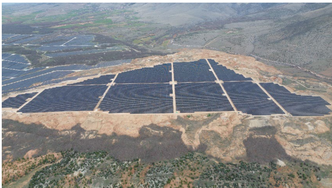
Figure 2: Section of a 171 MW photovoltaic plant located in a former deposition area of the Western Macedonia Lignite Center.
