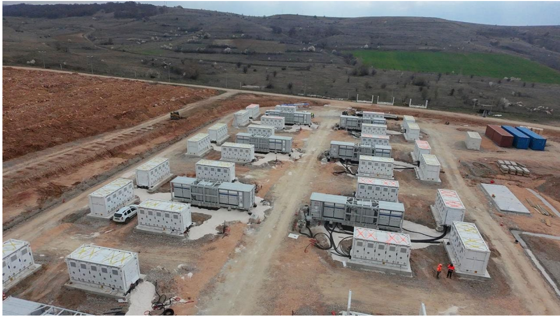
Figure 3: Battery array of the Meliti I Electrochemical Energy Storage Station.
