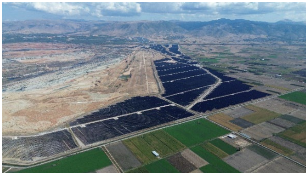
Figure 1: Part of a 550 MW photovoltaic facility located near the Agios Dimitrios Power Plant.
